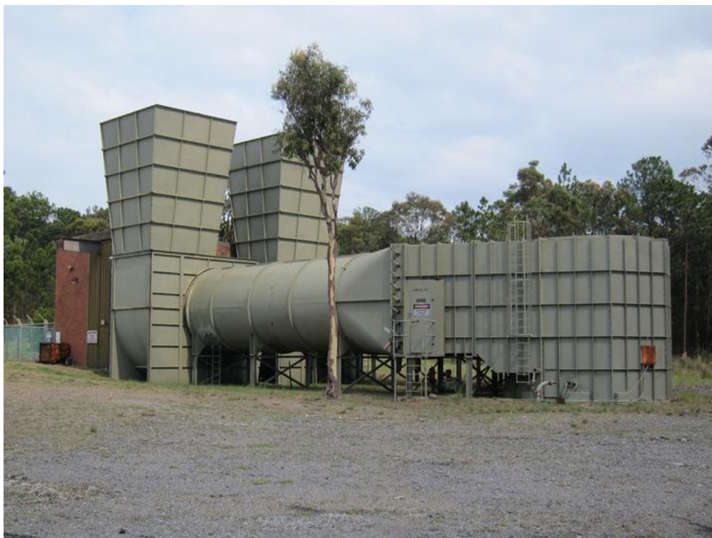
Plate 7.6: Mannering main ventilation fans
