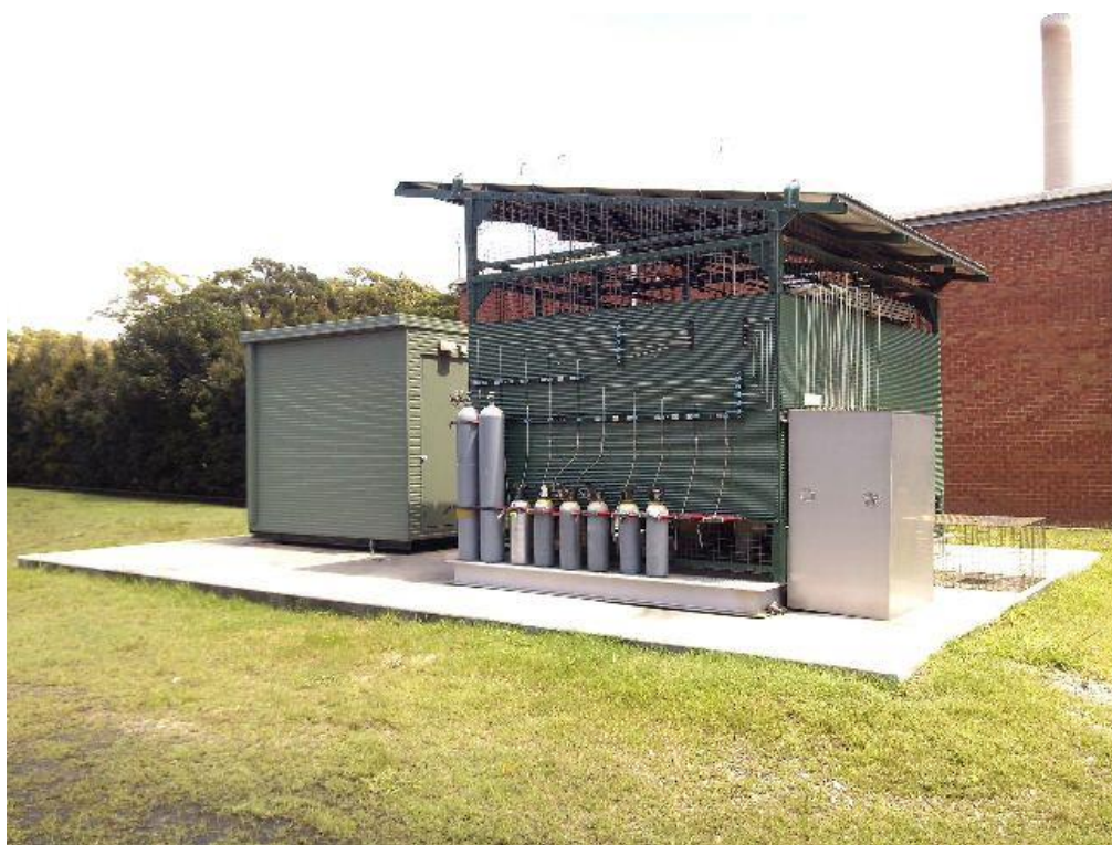
Plate 7.14: Chain Valley tube bundle monitoring (main winder and switchroom building behind)
